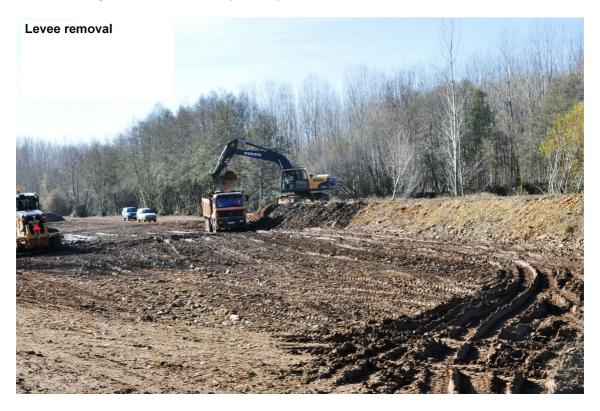
The project involved the naturalization of the river channel along a stretch about 24 km in length located in the upper section of the river. The actions consist of eliminating 8,710 m of levees and 4,720 m of rip-rap , moving away from the channel earth embankments and rip-rap along another 5,220 m, and recovering 10,063 m of secondary channels and adjacent fluvial areas. These actions
